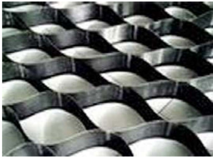
Figure 1 Typical geocell mattress, after [1]
