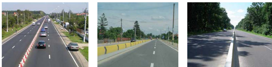
Figure 7 Safe median barriers
