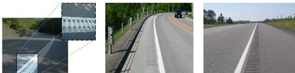
Figure 8 Shoulder rumble strips
