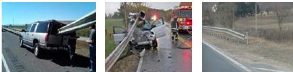
Figure 5 Unsafe barrier systems
