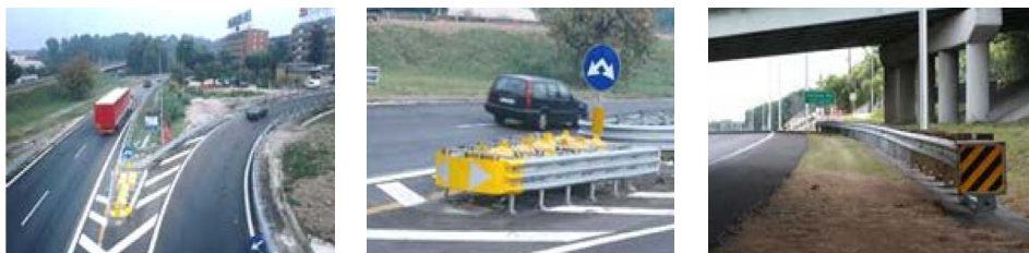
Figure 6 Safe barrier systems with proper ends
