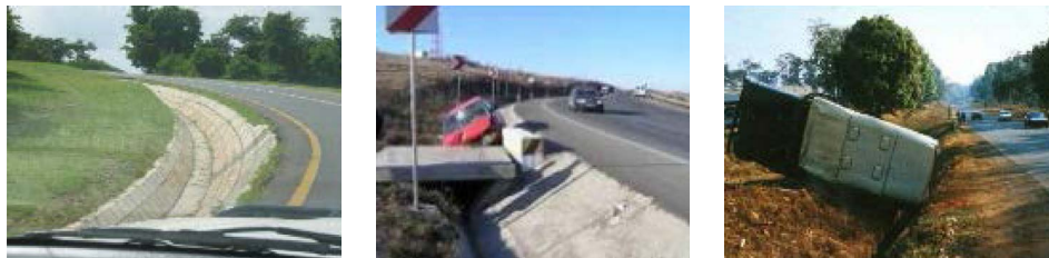
Figure 3 Unsafe drainage structures
