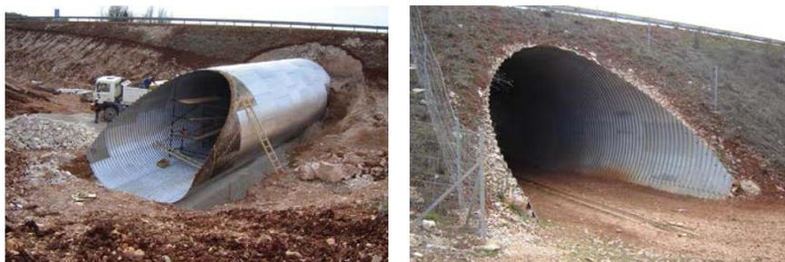
**Figure 9** Installation of animal underpass – phase II and animal underpass in km 5+030,00 of Adriatic Highway – ISTRIAN “Y”
