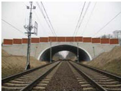
Figure 5 Animal overpass in Trzebaw (2002) (span of 17,68m) and above railway, Rzepin (2008); Poland
