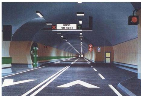
Figure 2 Example of properly installed traffic signs in a tunnel [3]
