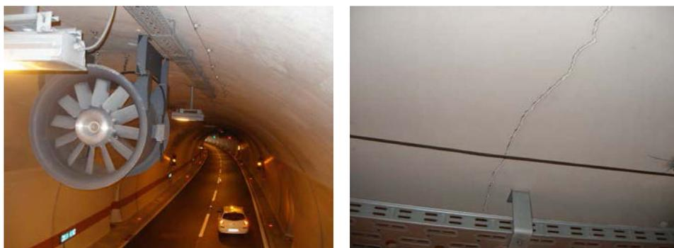
Figure 1 Crack in secondary concrete tunnel lining
