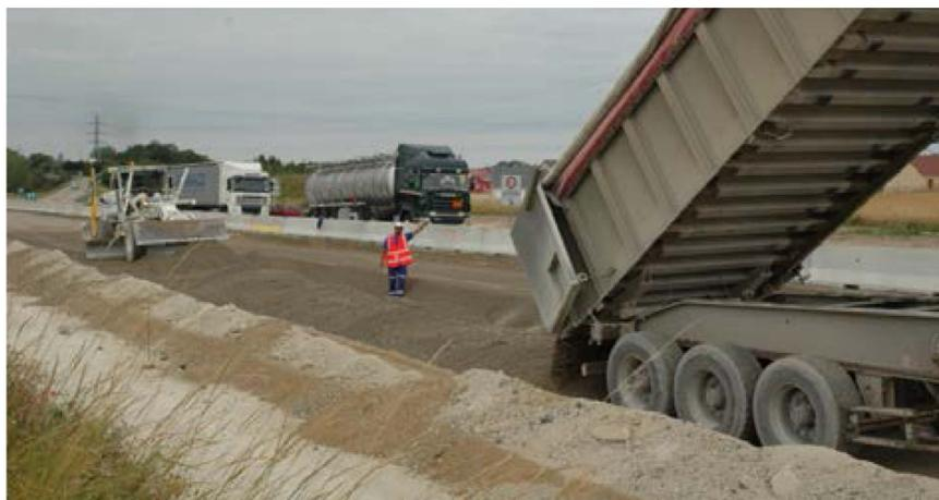
Figure 3 Laying of Recyvia® in the bypass of Troyes (France)
