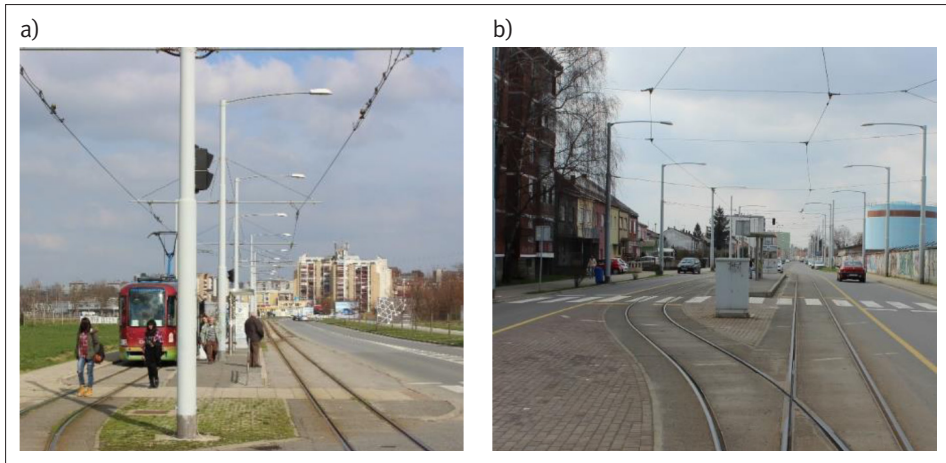
Figure 3 Tram stops: a) along the edge of the pavement, b) in the middle of pavement
