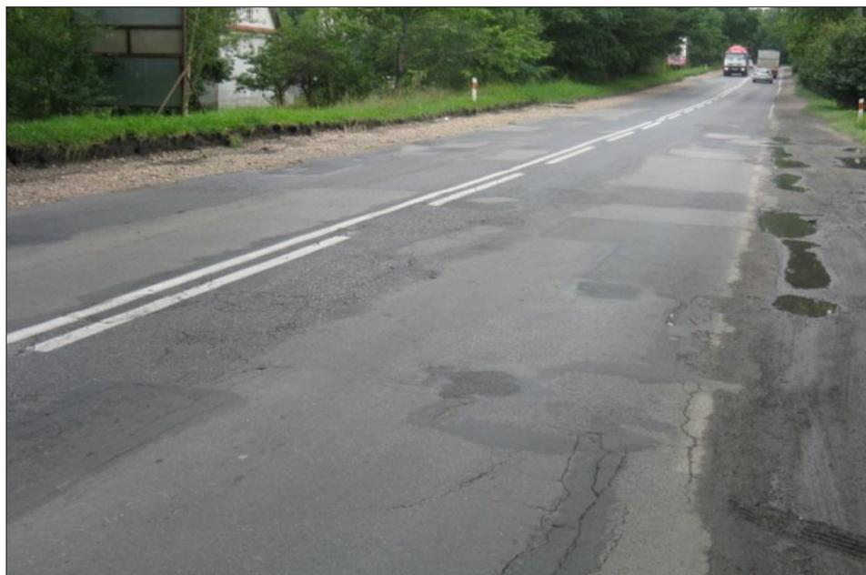
**Figure 2** View of damaged pavement on national road 44
