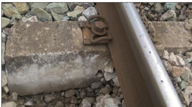
Figure 4 Replacement of ZEL.8 fastening with compatible fastening UTZ
