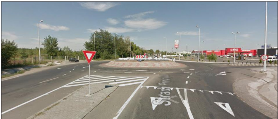
Figure 2 Example of roundabout with two lanes per direction
