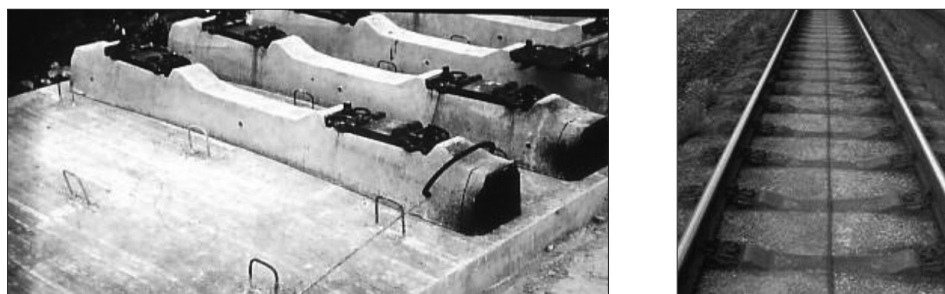
Figure 2 Test track at “Rheda” station during construction in 1972 (left) and today (right)
