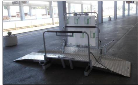
**Figure 8** Ramp for the disabled persons in the pedestrian underpass of the railway station Vinkovci and elevation platform
