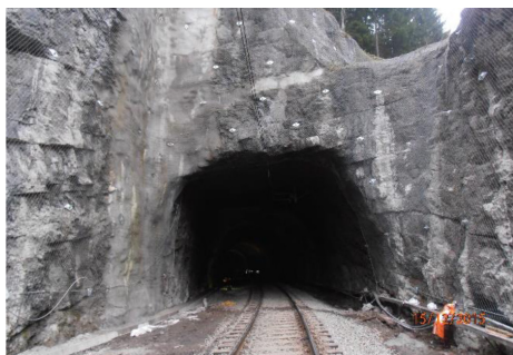
Figure 5 Cutting approach and entrance portal of the tunnel Kloštar and the rings at the exit part of the tunnel after reconstruction
