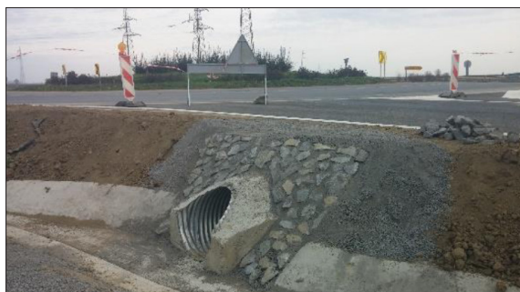
Figure 8 Completed culvert at roundabout entrance (first phase of construction) during construction work
