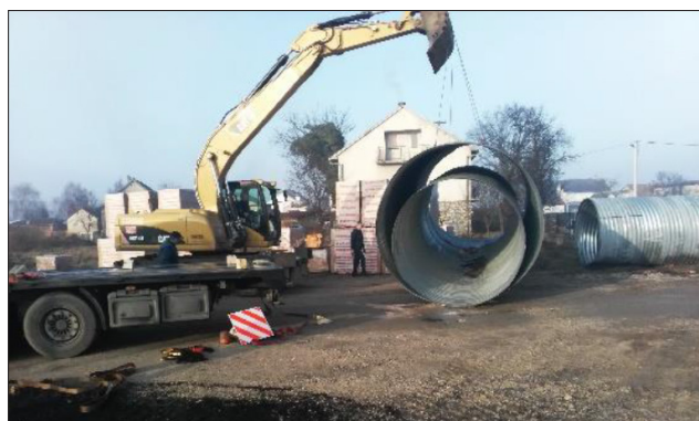
Figure 3 Transport and unloading of HelCor® spiral steel pipes
