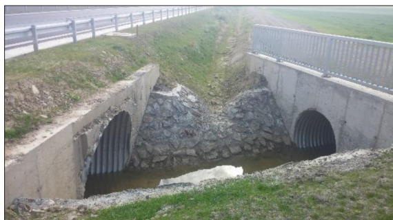
Figure 10 Culvert in road bed (HC 2000) and culvert in service road (HC 1600)
