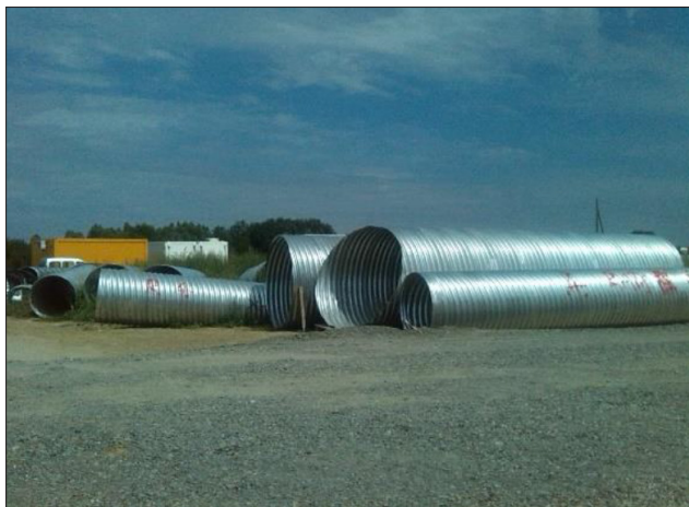
Figure 4 On-site storage of HelCor® spiral steel pipes
