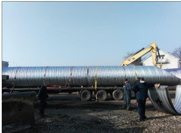
Figure 2 Transport of HelCor® spiral steel pipes
