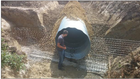
Figure 6 Both-sided backfilling with compaction and construction of walls
