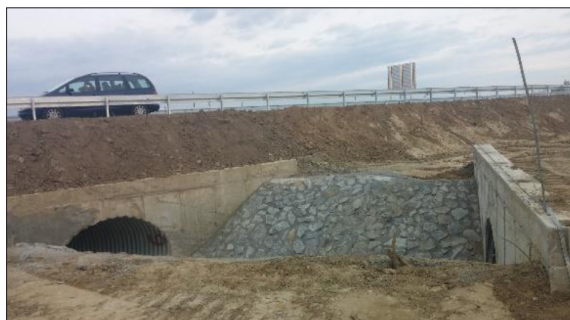
Figure 9 Culverts in use in road bed and service road
