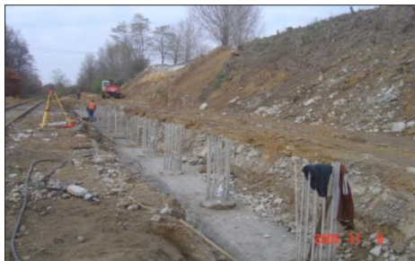
Figure 7 Supporting the soil-steel structure on a wall topping the piles
