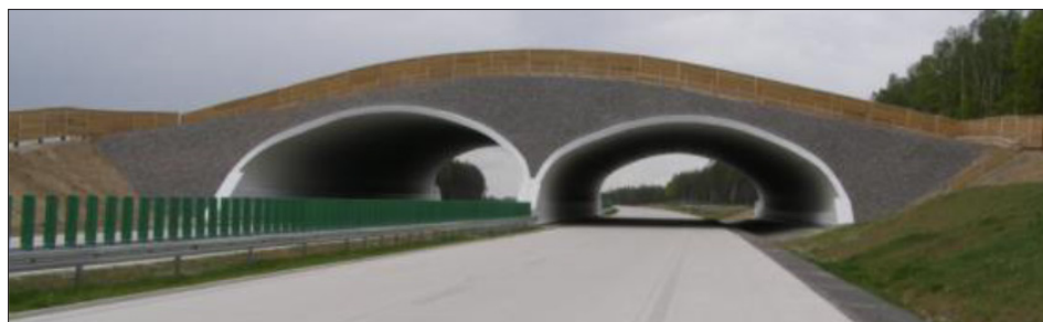
Figure 1 Central support of a twin soil-steel structure
