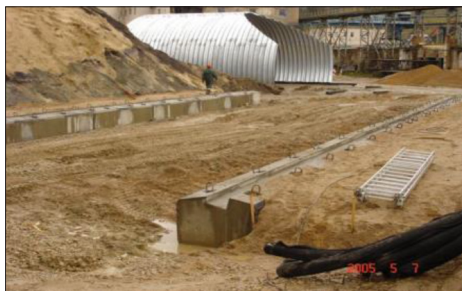
Figure 8 Supporting the soil-steel structures on piles
