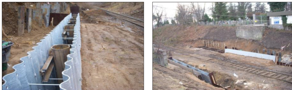
Figure 6 Supporting the soil-steel structures on piles
