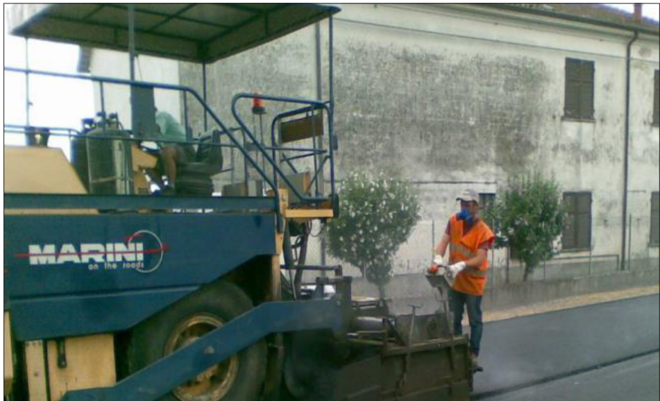
Figure 9 Laying of the wearing course
