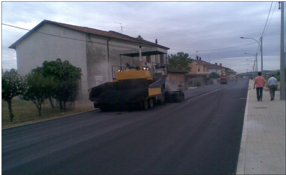
Figure 10 Laying of the wearing course and compaction with roller
