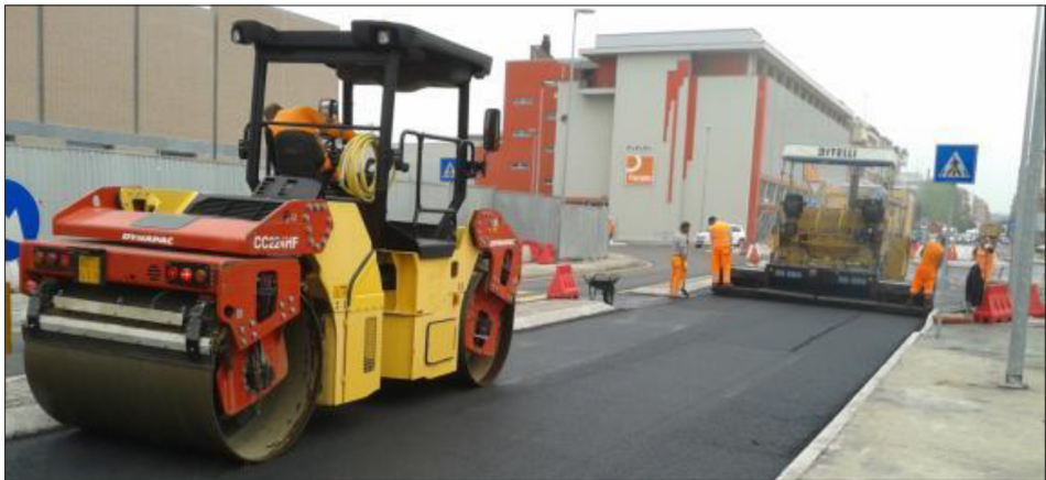
Figure 14 Laying of the wearing course and compaction with roller
