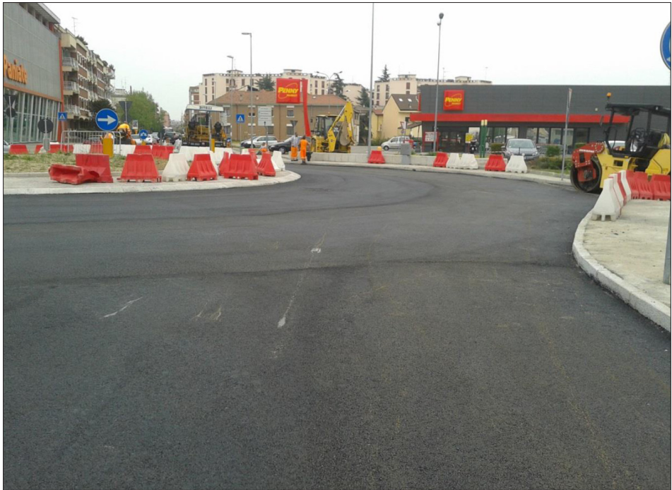
Figure 15 Wearing Course after compaction
