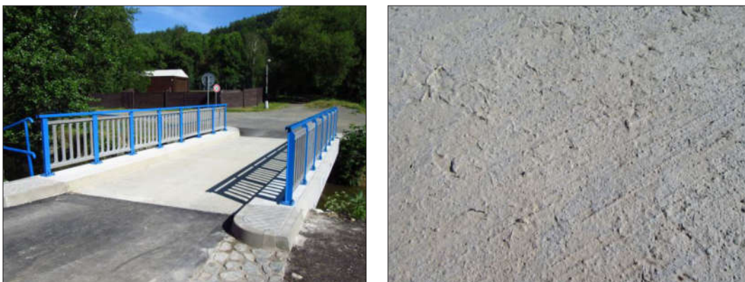
Figure 4 Left: The new bridge. Right: The surface of PFRC UCBD.
