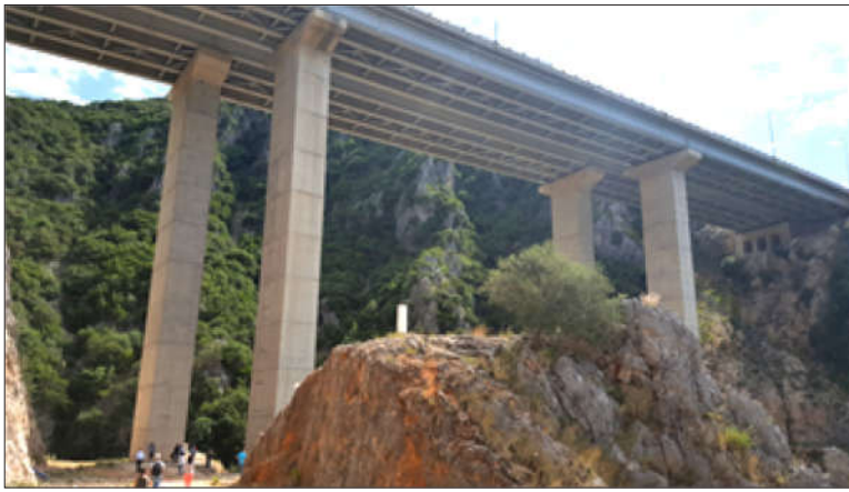
Figure 2 Egnatia Motorway G4 Bridge (© EOAE)
