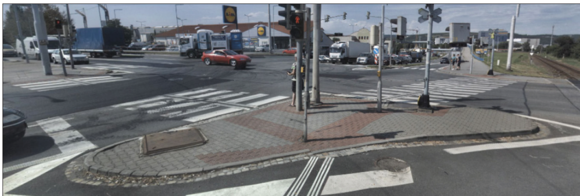
Figure 6 The dividing island does not meet the requirements about general technical requests ensuring barrier-free usage of constructions. The tactile line does not follow the signal and warning parts. People are led outside the pedestrian crossing into a wide and busy intersection. Further there are many obstacles on the island (difficult orientation) including insufficient waiting area.
