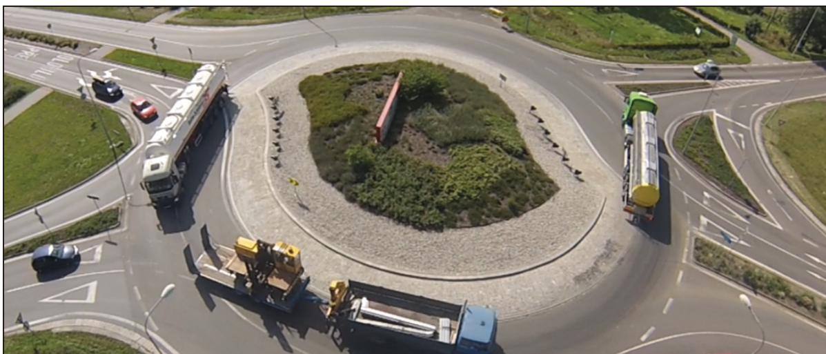
Figure 2 An example of observed conflict situation – passage of heavy lorry over two lanes (consequently other traffic participants are influenced). There is absent the physical separation of the lanes. Various serious situations were observed on this intersection. This intersection has an annual average of daily intensity of approx. 17 000 vehicle a day.
