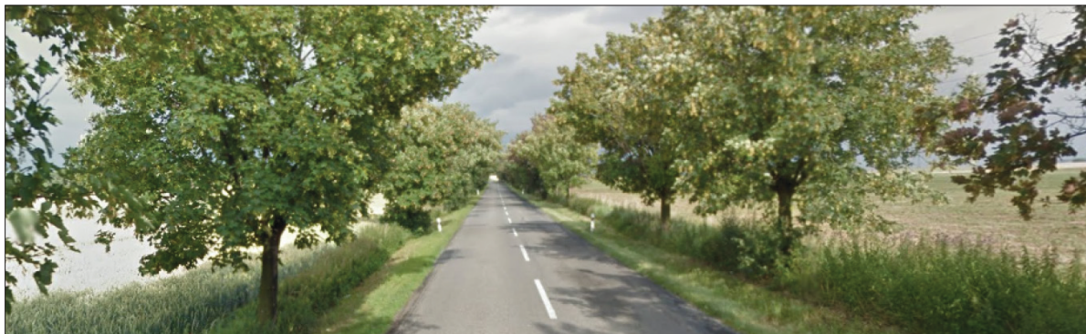
Figure 5 The fixed obstacle in the form of the roadside alley on the road of 2 nd class with an annual average of the daily intensity of approx. 5 000 vehicles a day. The trees are very close to the road, in some parts they are in very bad conditions and there is a danger of falling of the trees on the road. In this area there were 65 accidents with fixed obstacle (tree) in last 6 years. Two of them had a loss of a life as a consequence.
