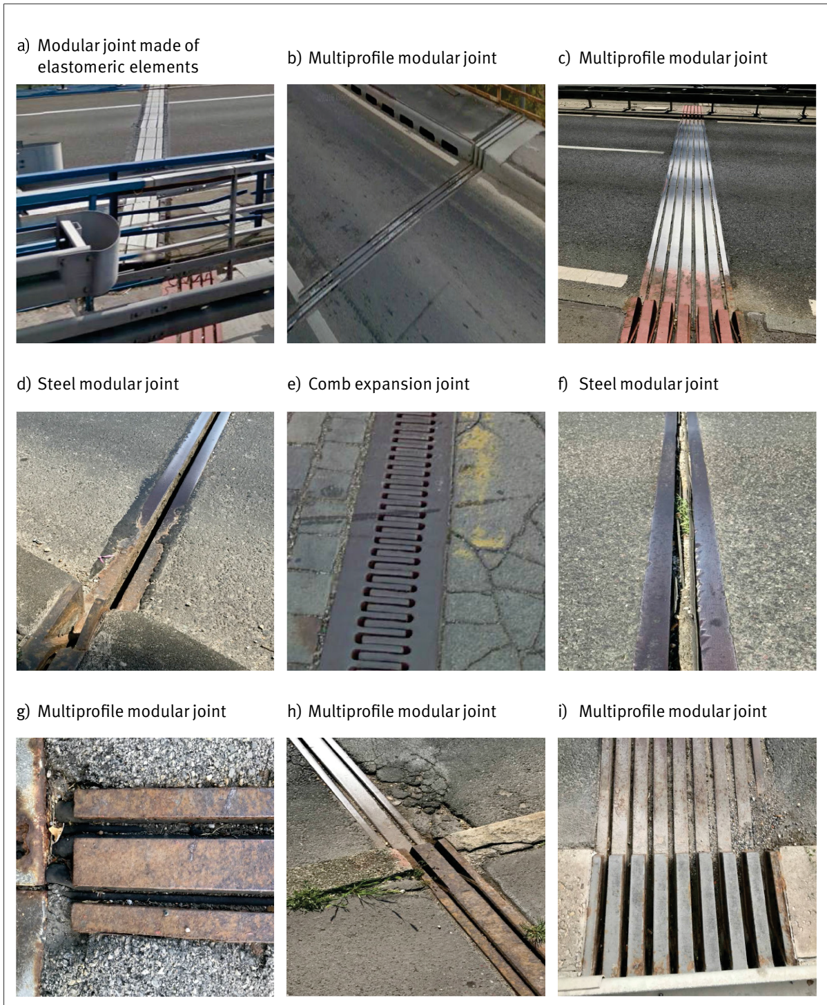
Figure 9 Examples of modular expansion joints on bridges across the Sava River in Zagreb: a) Zaprešić bridge; b) Podsused bridge; c) Jankomir bridge; d) Adriatic bridge; e) Sava pedestrian bridge; f) i g) Liberty bridge; h) Youth bridge; i) Homeland bridge
