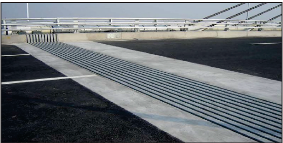
Figure 3 Multiprofile expansion joint with concrete hood [4]
