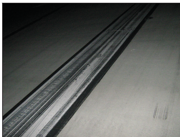
Figure 4 Pavement with marking on location A
