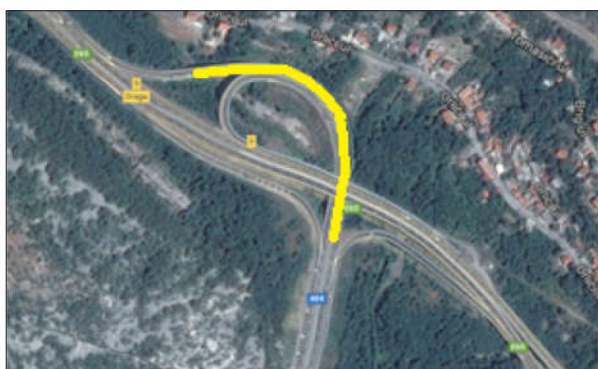
Figure 2 Junction Draga connecting state roads A7 and D404 with yellow marked analysed ramp
