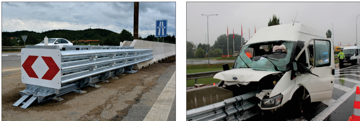
Figure 1 Crash cushion (left) [10] and traffic accident of the small truck on the D2 on October 2016 (right)
