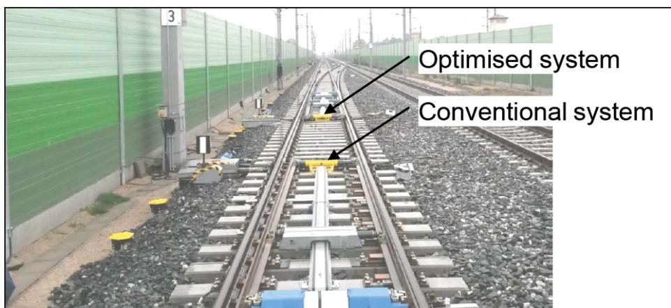
Figure 2 Selected points at a high-speed railway line in order to study the efficiency of the optimised and conventional heating systems for positioning systems contained in hollow sleepers
