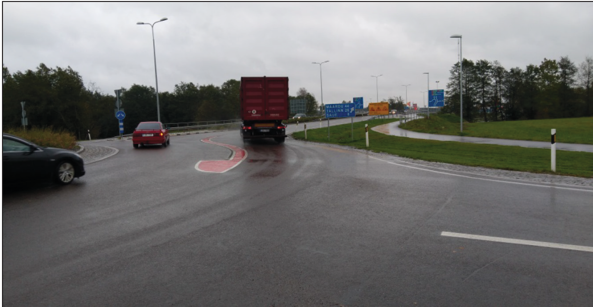
Figure 2 Example of the beginning of the divider for the spiral turboroundabout in Estonia
