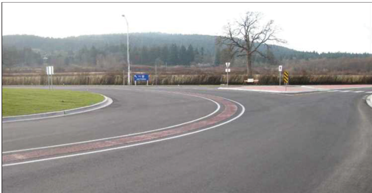
Figure 1 Example of the beginning of the divider for the spiral turboroundabout in Canada [1]
