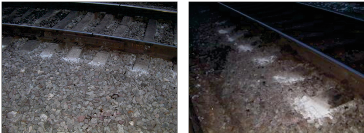
Figure 3 Visual control of trackbed vibrations in the case of adjustment by means of SB (left) and TM (right)
