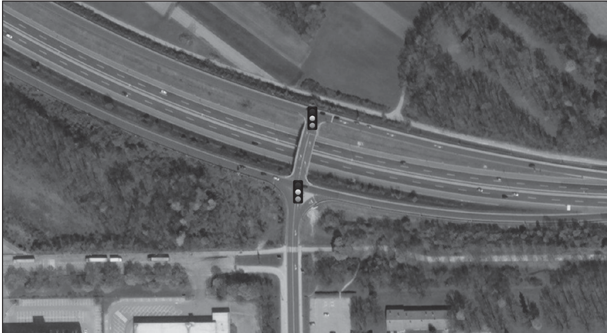
Figure 3 Existing situation at Leskovškova cesta
