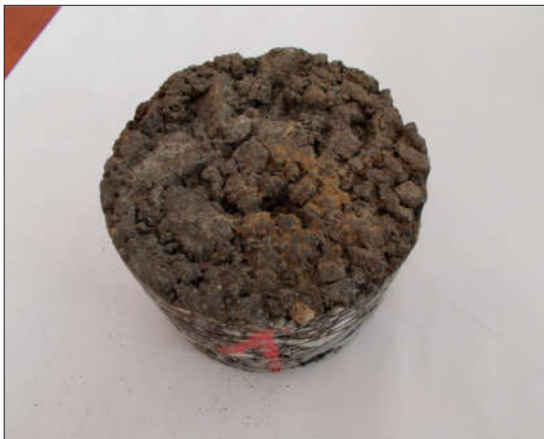
Figure 3 Asphalt core sample from affected area
