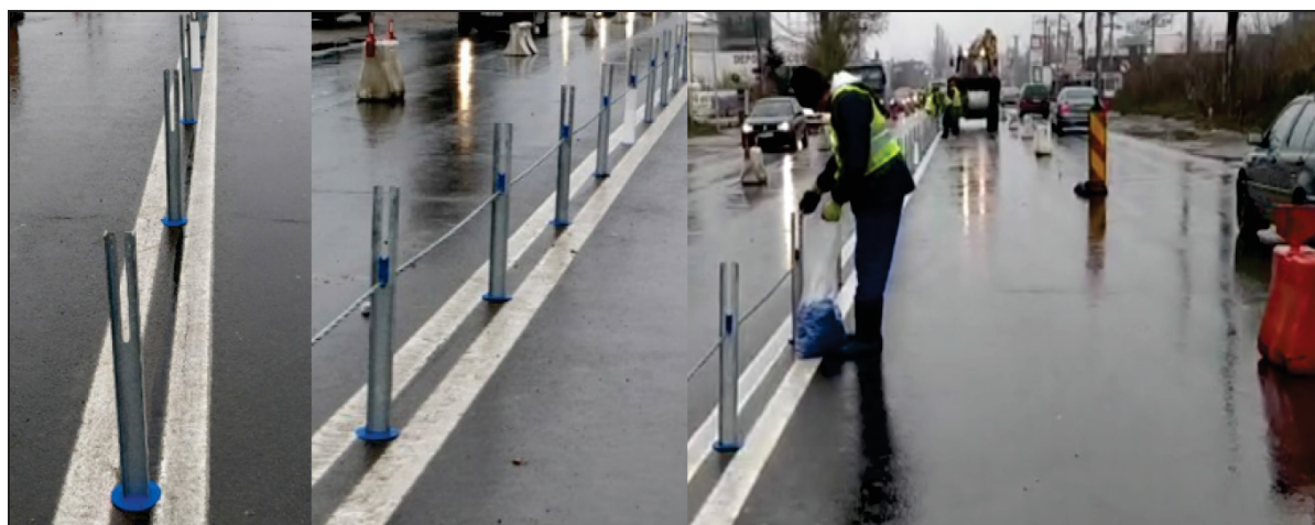
Figure 7 Mounting the cable barriers
