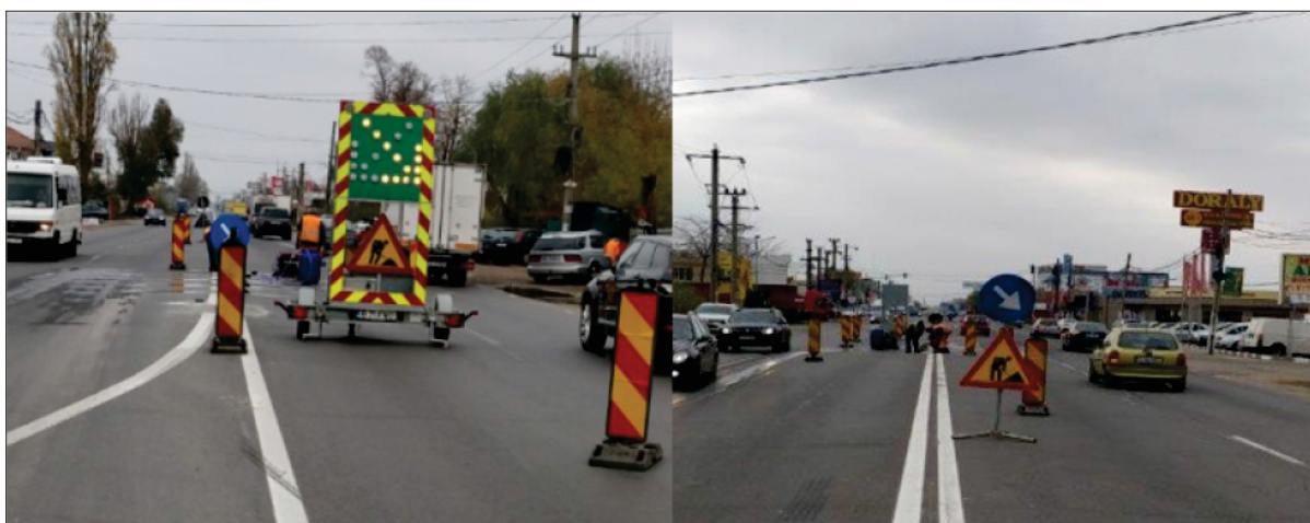
Figure 5 Temporary road signaling
