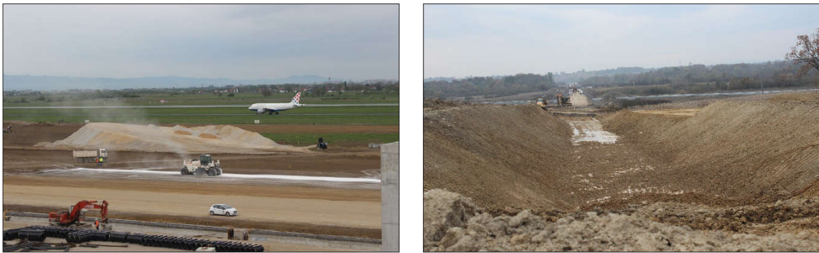
Figure 2 Subgrade construction sites of airport (left) and railway (right)
