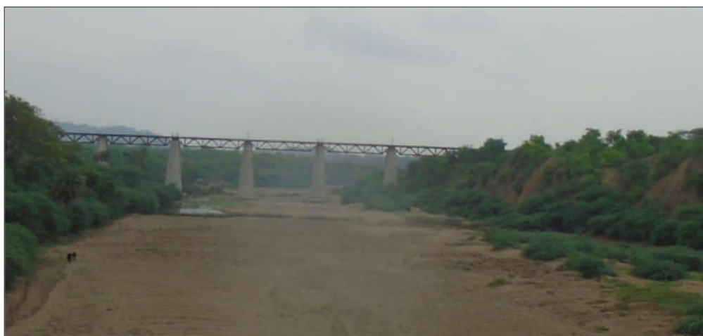
Figure 5 View of the existing Indian Railway Bridge
