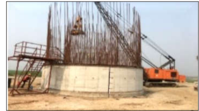
k) Mucking & Sinking Arr. & ready for next lift (on site activities)
