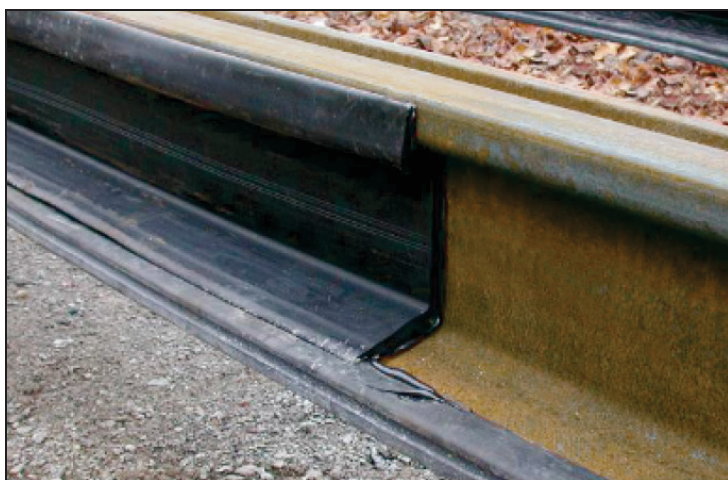
Figure 4 Rail boot placed on whole length of the rails, [24]
