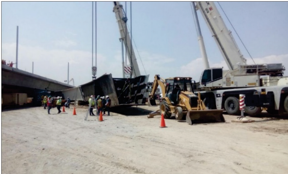
Figure 11 Viaduct 6 during the final stages of assembly
