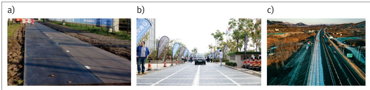
Figure 6 Solar road: a) the trial segment of a solar road [30], b) the first photovoltaic pilot zone in China, in the city of Jinan, Shandong district [31], c) solar power highway [32]
