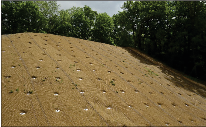
Figure 13 Evenly profiled embankment in loose rock with close-fitting erosion protection mat
