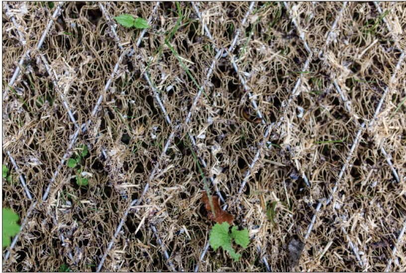
Figure 14 TECCO® GREEN after hydroseeding
