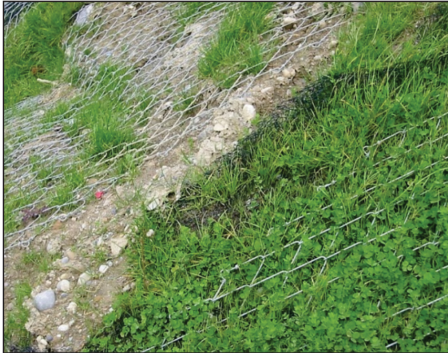
Figure 9 Test area approx. 10 weeks after the hydroseeding process and after heavy rainfall. On the left the reference surface without an erosion protection mat with less than 10 % greening success. On the right with a geomat and a greening success of more than 90 %
