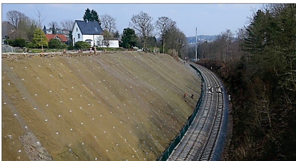
Figure 12 Securing a cut slope after a landslide in the weathered rock
