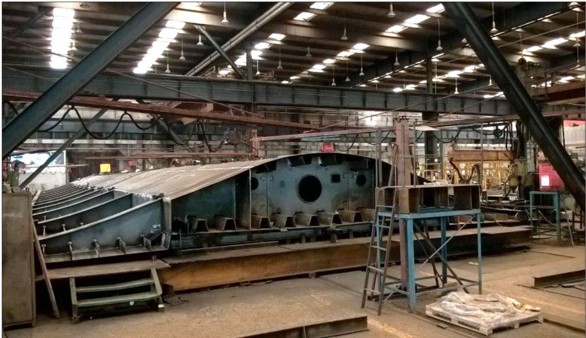
Figure 8 Execution of orthotropic deck box girder superstructure segments in the workshop
