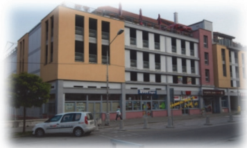
Figure 2 Trenčín - parking house
