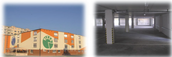
Figure 1 Parking house in Zvolen – housing estate Západ
