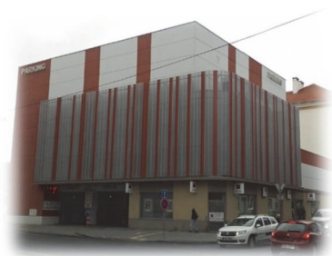
Figure 5 Parking house with APS in Slaný
