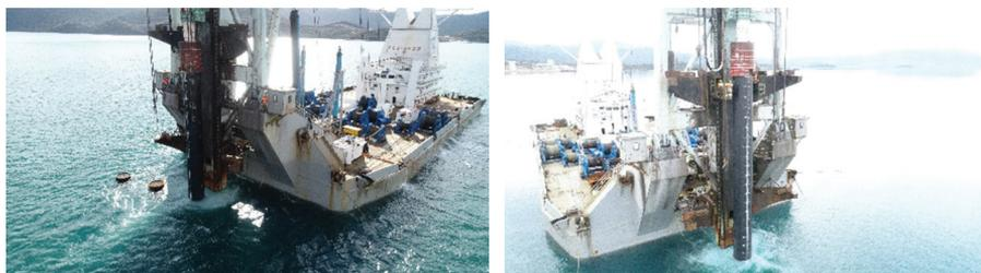
Figure 3 Steel pile driving by large-scale driving barge
