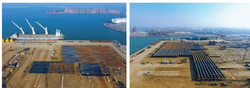
Figure 2 Steel tubular piles storage at port and uploading to cargo vessel
