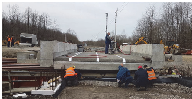
Figure 4 Reinforced concrete span structure of the bridge
