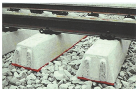
Figure 6 Elastic beddings under the concrete sleeper [1]
