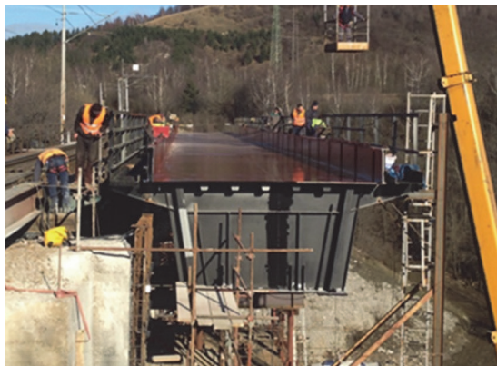
Figure 3 Steel structure of the bridge
