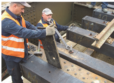
Figure 2 Attaching wooden sleepers to the steel structure of the bridge
