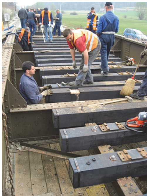
Figure 1 Individual processing of wooden sleepers on a steel bridge
