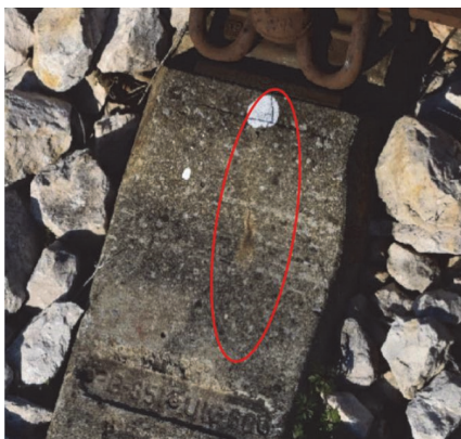
Figure 4 TYPE 1 cracking
