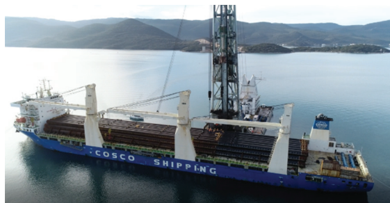
Figure 4 Cargo vessel with extra-long steel piles arrival on site
