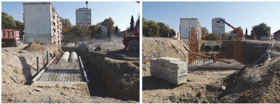
Figure 6 Leaking pipes for the hot water pipeline on Remetinečka cesta
