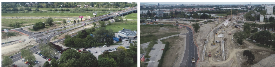
Figure 9 Temporary traffic management during the works
