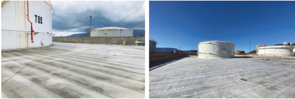
Figure 4 Concrete Canvas Hydro after 28 days
