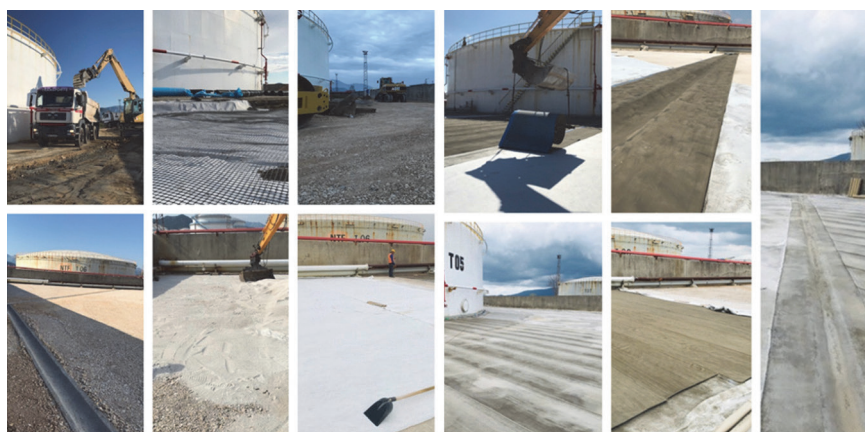
Figure 3 Step by step Concrete Canvas Hydro installation
