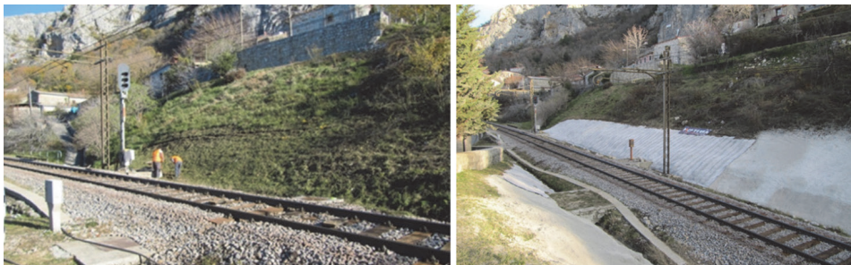
Figure 5 Slope before fire protection (left), slope after fire protection (right)
