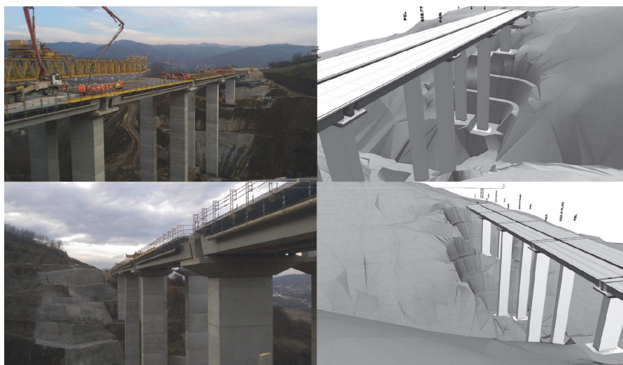
Figure 8 Bridge on site vs virtual bridge (BIM model)
