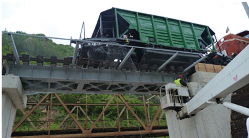
Figure 5 Static load test of the temporary railway bridge
