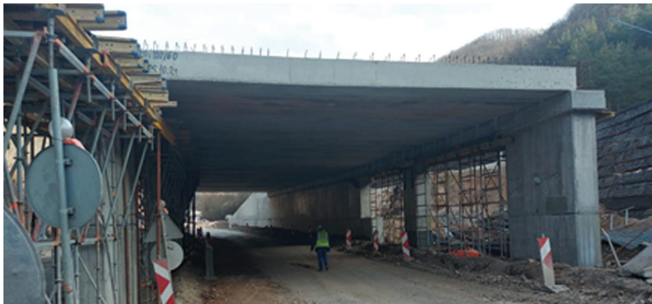
Figure 9 The structure of the new railway bridge is almost completed
