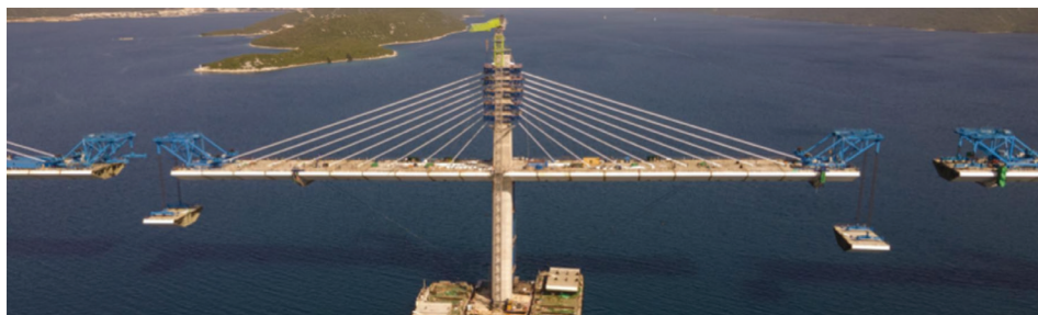
Figure 7 Standard segments installation with by derrick cranes (June 2021) Credit: CRBC
