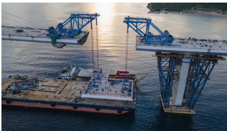
Figure 3 The first closure segment CR4 (29.7m long) installation (June 2021) Credit:CRBC
