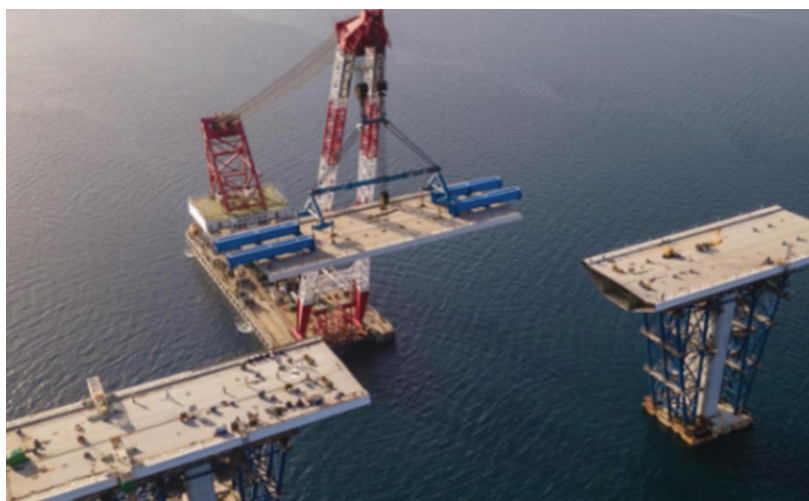
Figure 8 Extra-large segment R11 installation by 1000t floating crane (June 2021) Credit: CRBC
