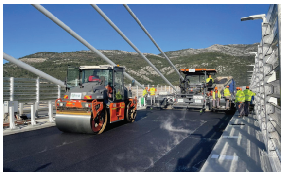
Figure 5 Wearing layer AC11S construction (Jan.2022) Credit: CRBC
