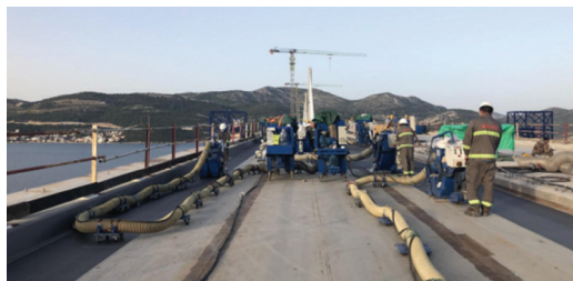
Figure 2 Shot blasting construction (September, 2021) Credit: CRBC
