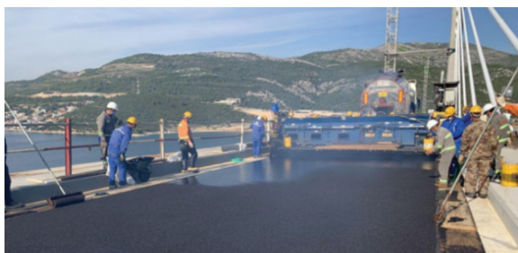
Figure 4 Mastic asphalt MA11S pavement construction (November 2021) Credit: CRBC
