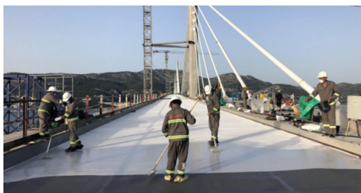
Figure 3 The epoxy resin waterproofing system construction (October, 2021) Credit: CRBC
