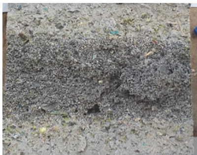
Figure 6 Cross-section of the beam where the inhomogeneous core is clearly visible
