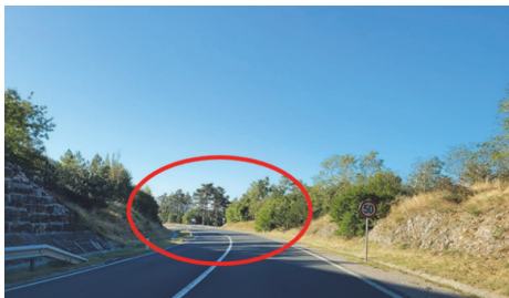
Figure 2 Bad visibility of the roundabout and stopping sight distance [1]
