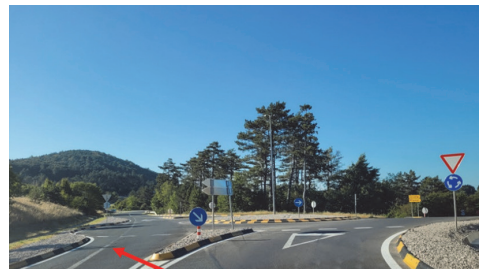
Figure 3 Old misleading centerline [1]
